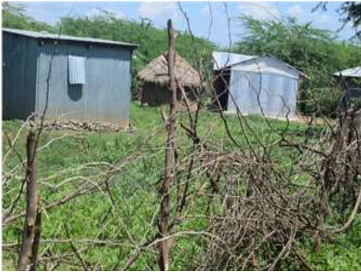
Plate 7: House constructed by Red Cross
